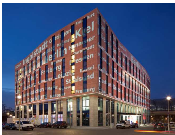
Completed in 2013: InterCityHotel near the Berlin main railway station
