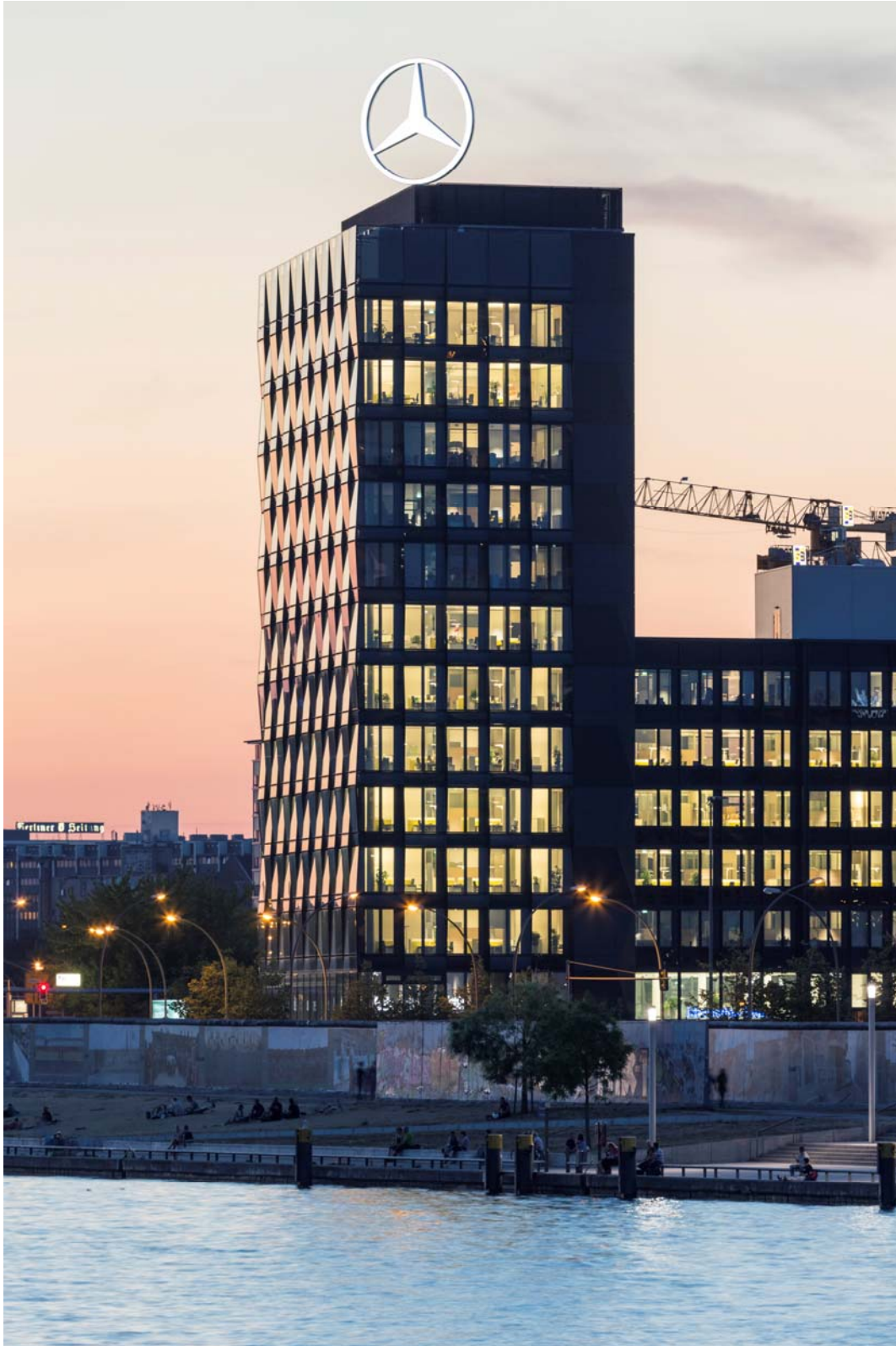
Mercedes-Benz sales division Germany: Completion and hand over to tenant in mid-July 2013
