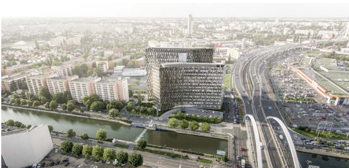
Visualisation of the office project Orhideea Towers in Bucharest
