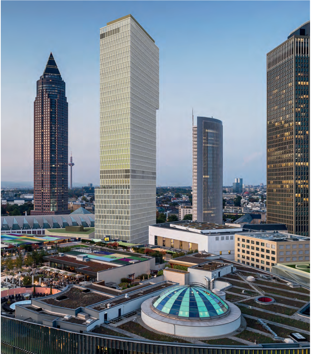
CA Immo is developing the office and hotel high-rise ONE between the Frankfurt banking district, exhibition center and the Europaviertel
