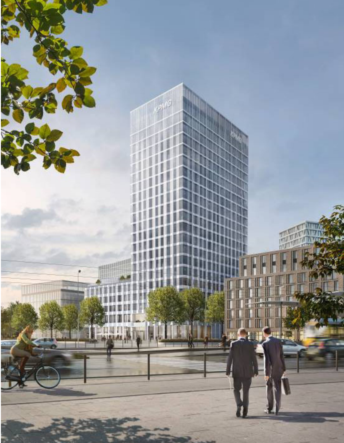
In Berlin CA Immo is currently constructing the High-rise Building on Europaplatz.
