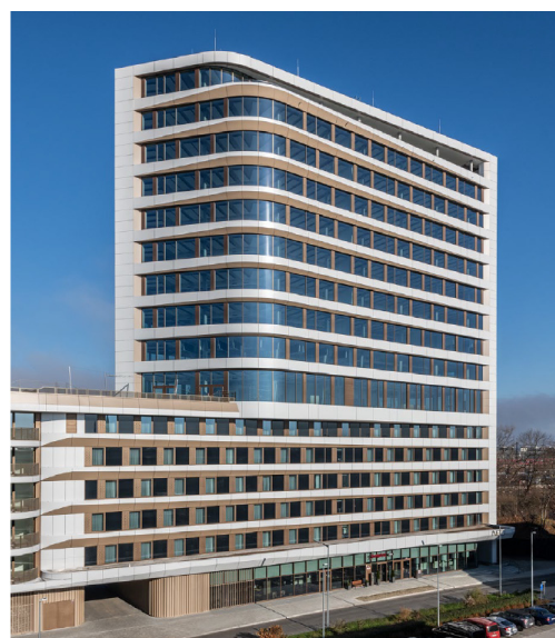
Completed in 2020 and part of the CA Immo investment portfolio: NEO office building, Munich
