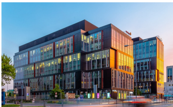
Part of the CA Immo portfolio since the end of October: the Warsaw office building Postepu 14
