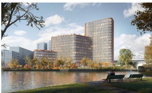
100% pre-let: Upbeat office tower near Berlin Central Station
