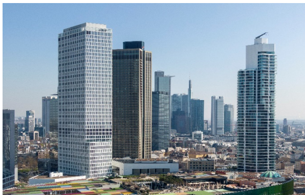
The ONE in Frankfurt (left), was the first high-rise in Germany to receive WiredScore Platinum certification for best connectivity.
