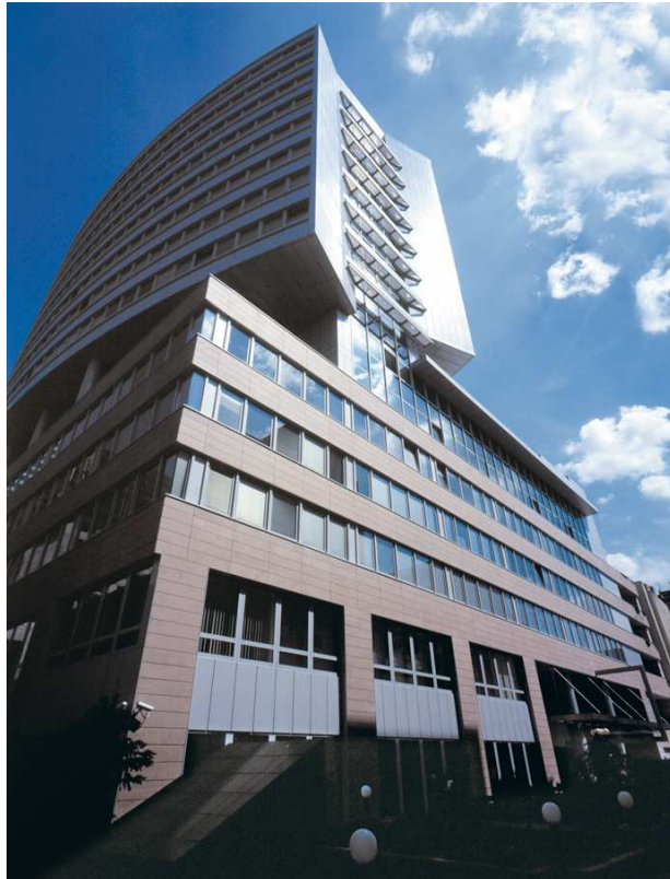
Warsaw Towers (21.000 m 2 , € 72 m, 7.1 %)
