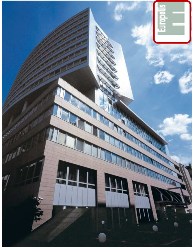
Warsaw Towers (21.000 m 2 , € 72 m, 7.1 %)
