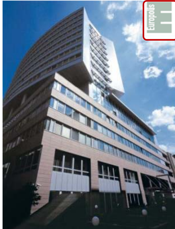
Warsaw Towers (21.000 m 2 , € 76 m)
