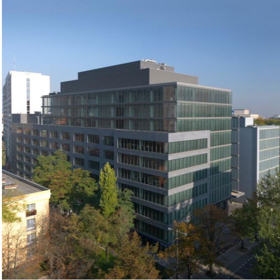
Saski Crescent, Warsaw
